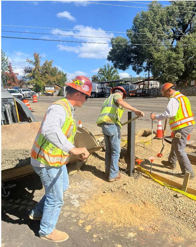
Installing posts for chain railing
